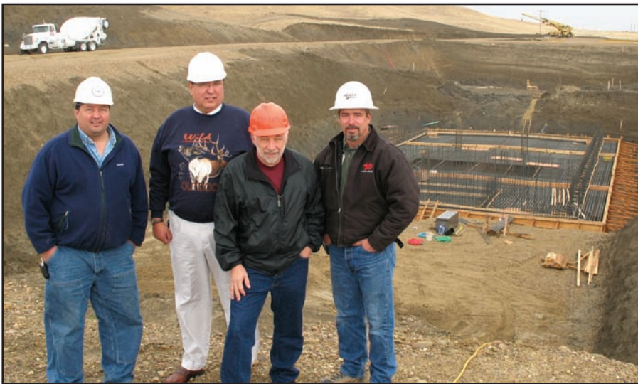
Fort Peck's Water Purification Plant under construction by Apollo on the Reservation. From left: Brian Boland, Field Rep, Montana Laborers Union; Kevin Buckles, TERO Director, Fort Peck Tribes; Ed Hensley, Construction Market Representative, LECET; Ron Harris, Project Leader, Apollo, Inc.
