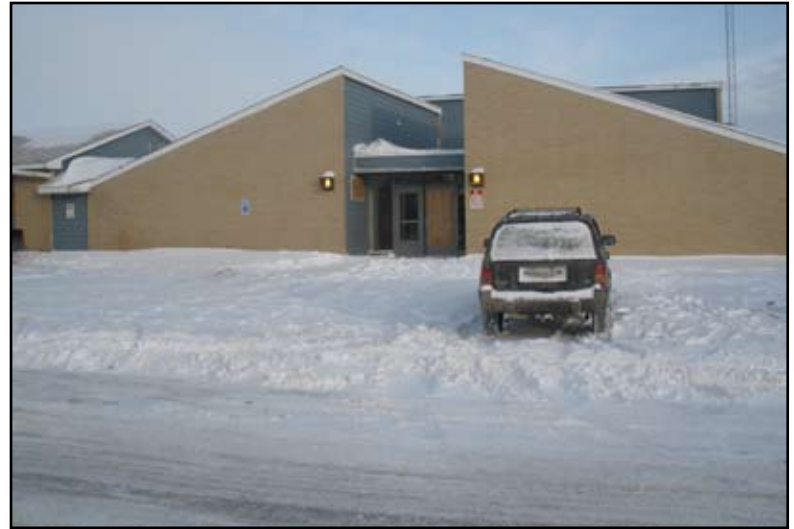
Commercial Building being renovated by NCCI class at Spirit Lake, ND
